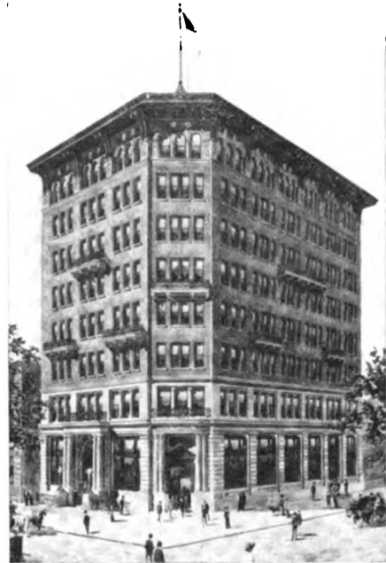
NEW HOME OF THE PEOPLE'S NATIONAL BANK, CHARLESTON, S. C.
